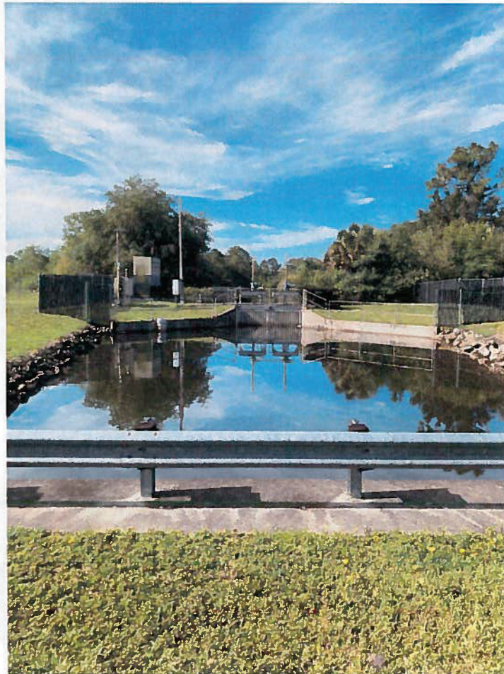
Figure 34 – Control No. 1 Pump Station
