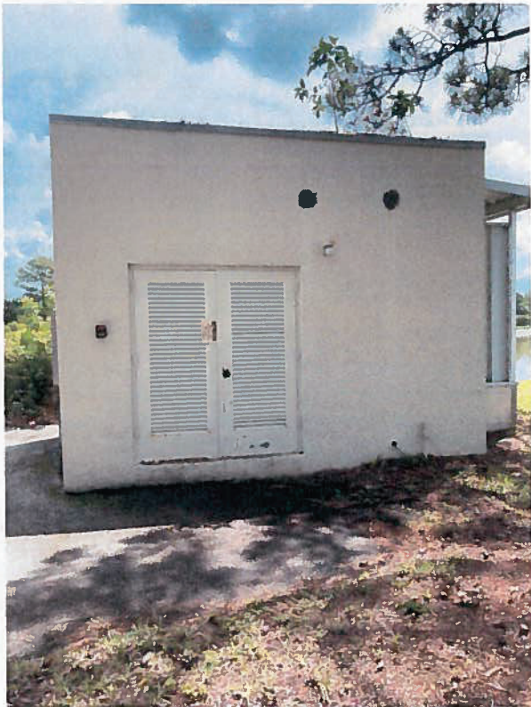
Figure 44 – Irrigation Pump Building
