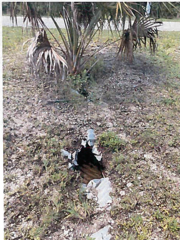
Figure 32 – North end of 12” CMP culvert under Innovation Drive
