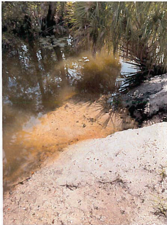
Figure 24 – Sediment washed into north canal at repair area
