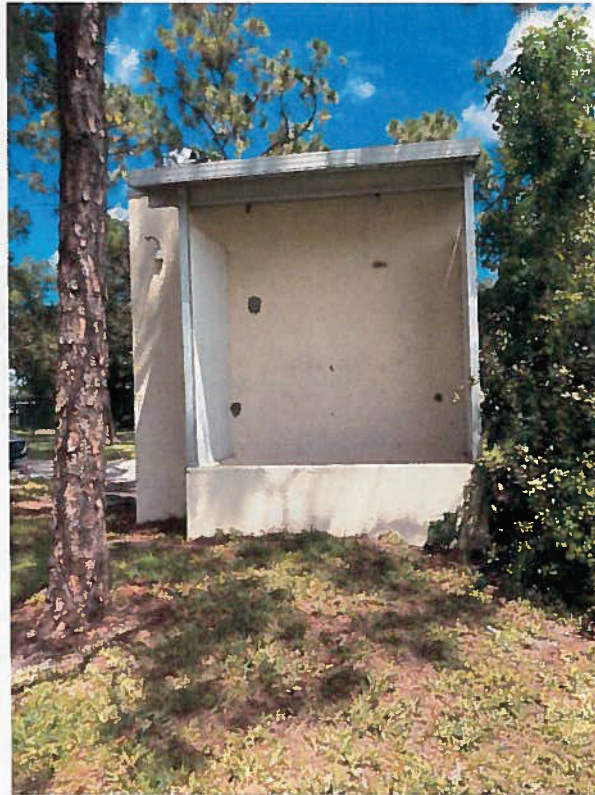
Figure 46 – Former fuel tank location at pump building
