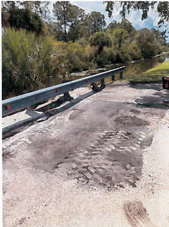
Figure 22 – Parking area west of FPL recently repaired along north canal
