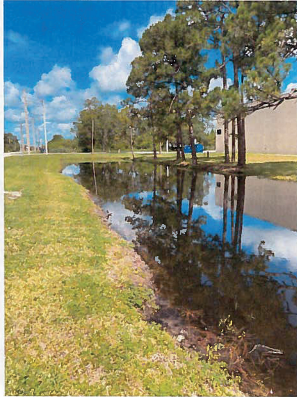
Figure 10 – Looking west at canal on north side of Innovation Drive
