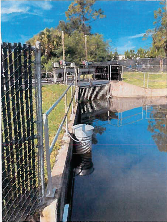
Figure 36 – Stilling well at Control No. 1
