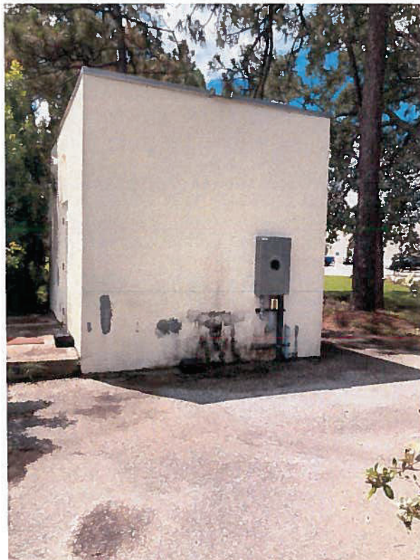
Figure 47 – Irrigation pump building
