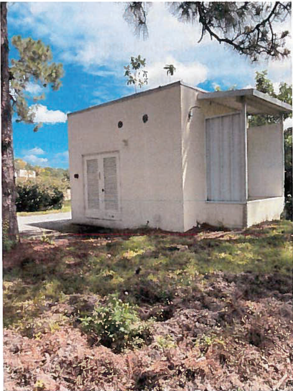
Figure 45 – Irrigation Pump Building
