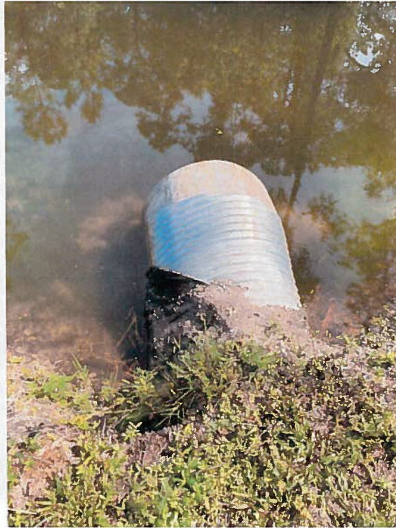
Figure 16 – South end of slip-lined culvert under Innovation Drive
