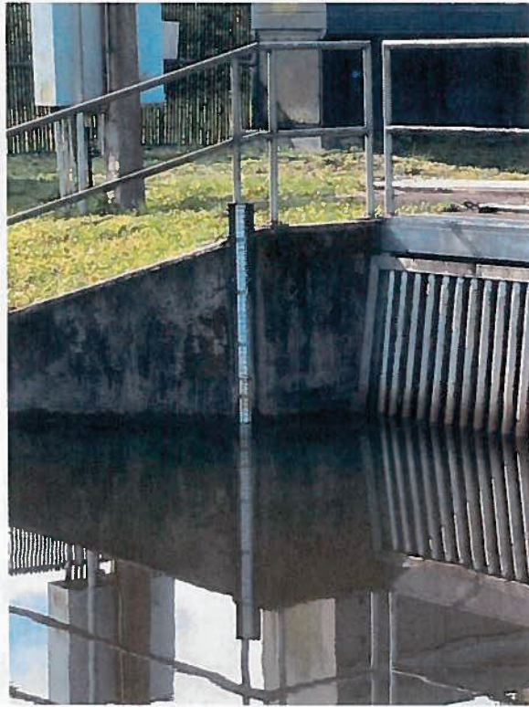
Figure 41 – Staff gauge at Control Structure No. 1
