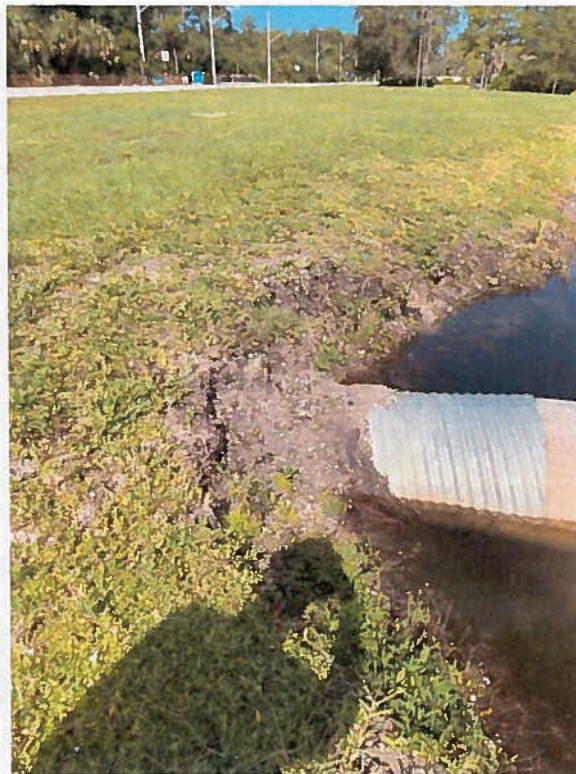
Figure 15 – North end of slip-lined culvert under Innovation Drive
