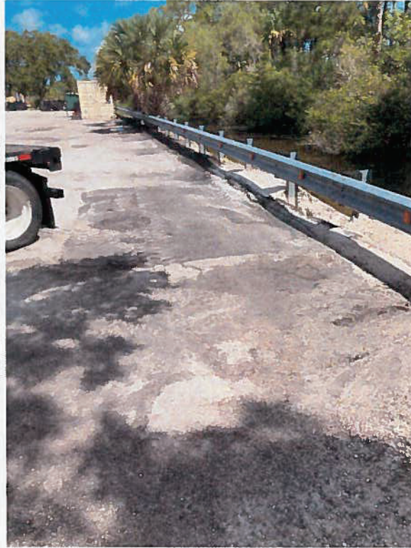
Figure 21 – Parking area west of FPL recently repaired along north canal
