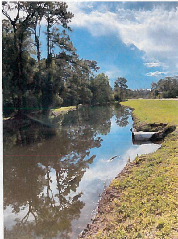
Figure 13 – North end of lined culvert under Innovation Drive
