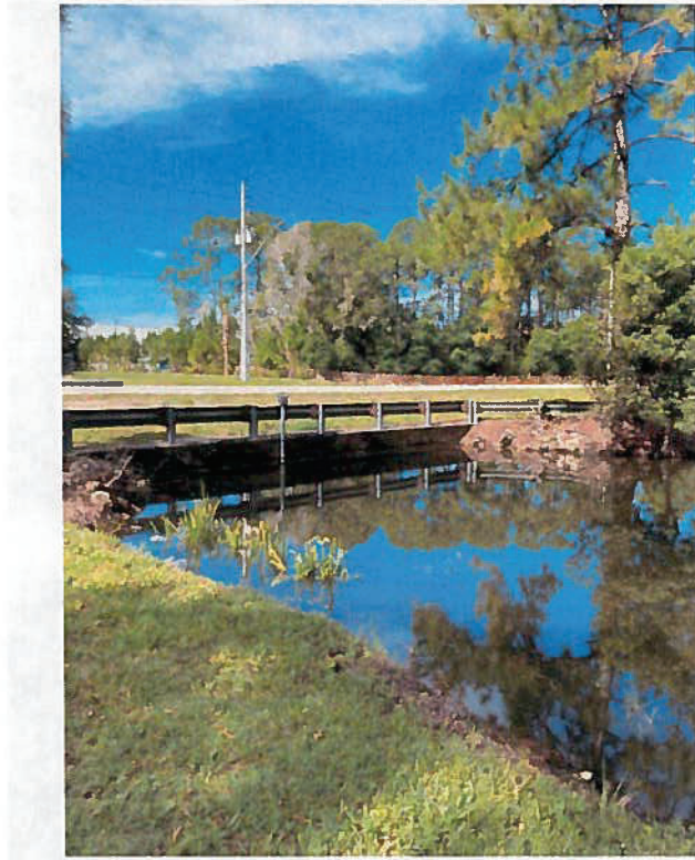
Figure 12 – Looking south at outfall canal upstream of Innovation Drive
