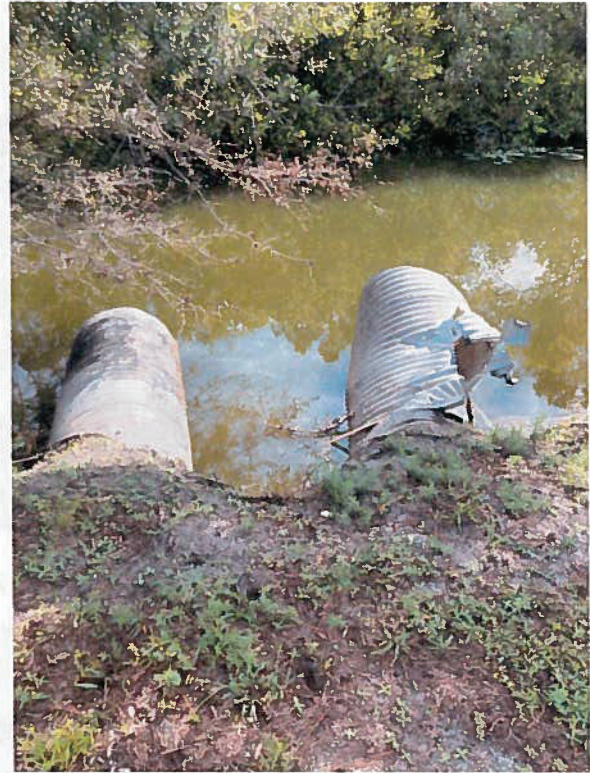
Figure 30 – Overflow Culverts from Stormwater Tract to North Canal
