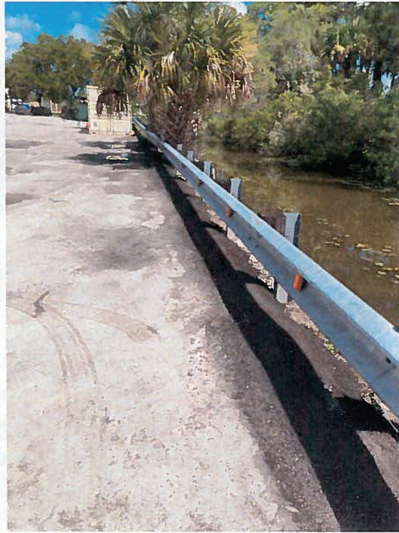
Figure 23 – Asphalt added along guardrail
